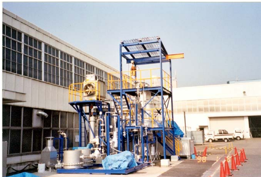
Figure 5.1: Photograph of the gasifier installation at Hiroshima
