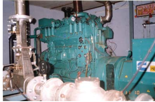
Plate 9.3 Gas engine with indigenous gas carburetor
