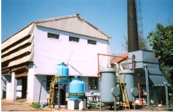
Plate 9.2 Overview of the gasifier plant at Metupalyam
