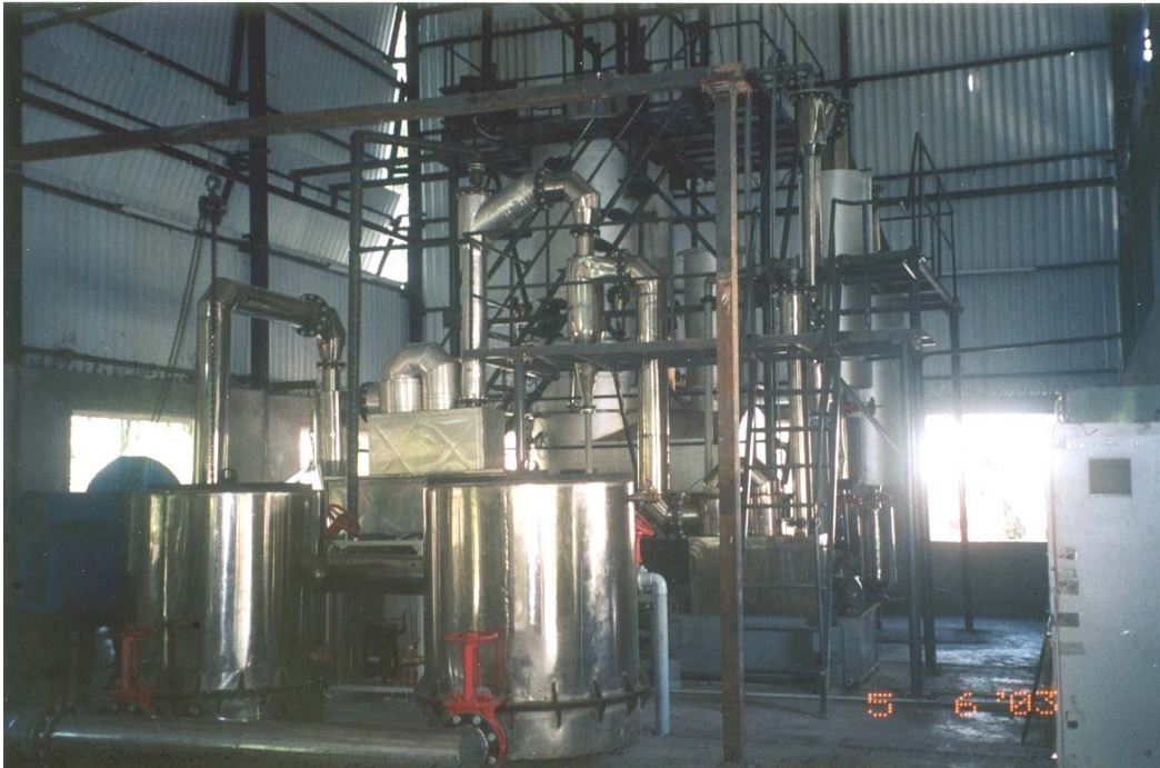
Plate 8: Gasification Plant at M/S Hindustan Pencils
