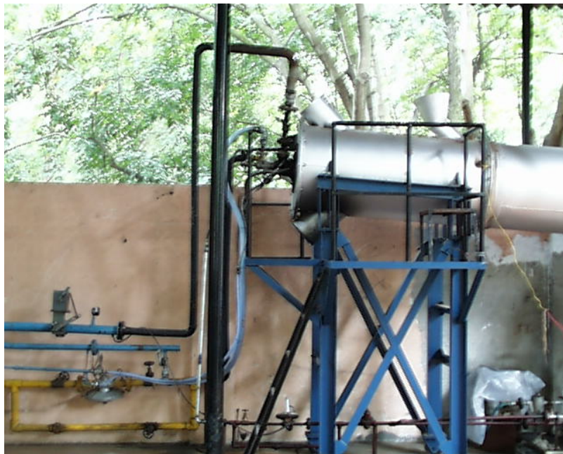
Plate 3.3: Feed inlet and Combustion Chamber of Rotary Drier.
