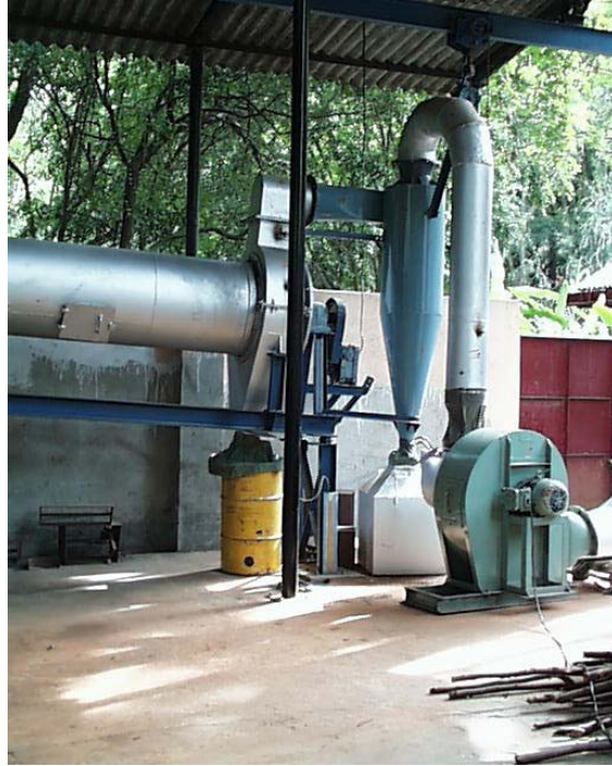
Plate 3.2: ID Blower and Cyclone attached to the Rotary Drier
